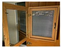
outer door to provide a finger grip and installed rare earth magnets to hold the door closed – very clever and functional features of this original design.
